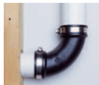
The extra length of the Qwik Ell completes the repair
