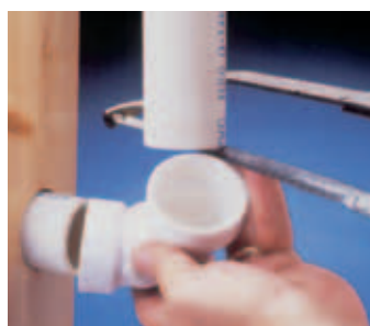
Damaged or leaking fitting is cut out
